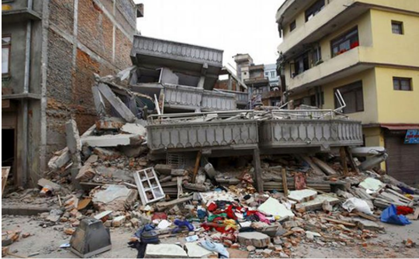
Photo 5: Wreckage from June 2015 Malaysia Earthquake
