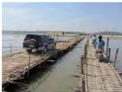
Temporary bridge at the affected site (Pauk Township)
