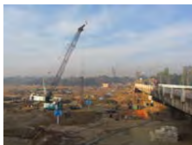
Construction of new Shwe Chaung Bridge (Pakokku Township)
