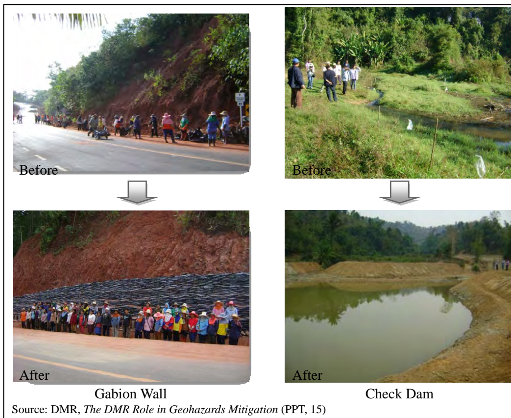
Figure 6.4.7 Countermeasures against Landslide
