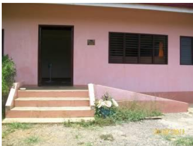
Accessible evacuation center
