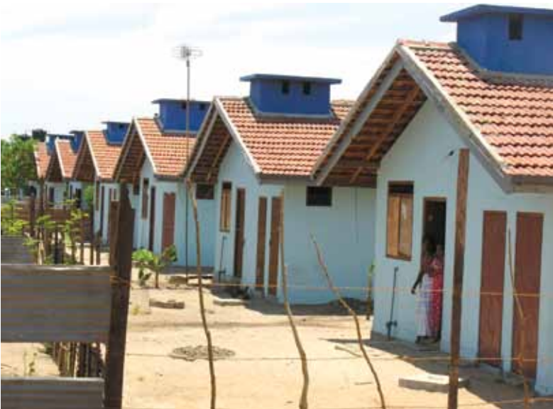
New homes in Batticaloa – The Red Cross helped to build over 30,000 houses during the five year tsunami recovery operation
